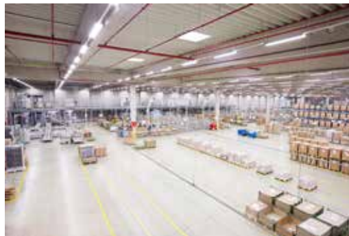
Hettich logistics center.
